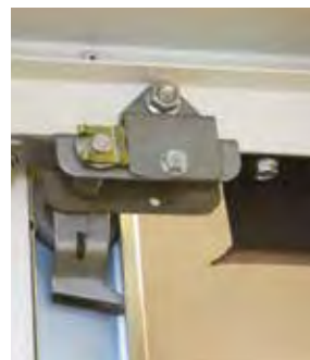
Anti drop mechanism. Large spindle roller. Spindle roller bracket has a reinforcement bracket to stop excessive movement.
