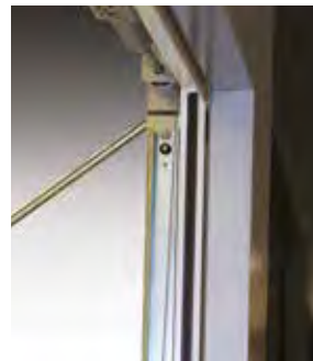
Anti drop mechanism. Large spindle roller. Spindle roller bracket has a reinforcement bracket to stop excessive movement.
